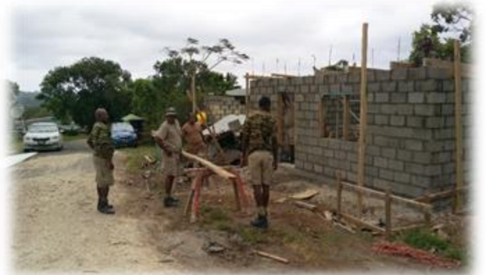
Rebuilding Cooks Barrack Coop through DFAT Pam Recovery
